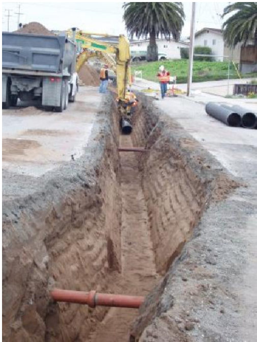
CRESCENT AVENUE CONSTRUCTION #3
