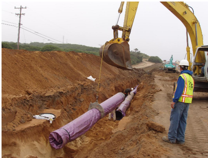
GENERAL JIM MOORE BOULEVARD CONSTRUCTION #2
