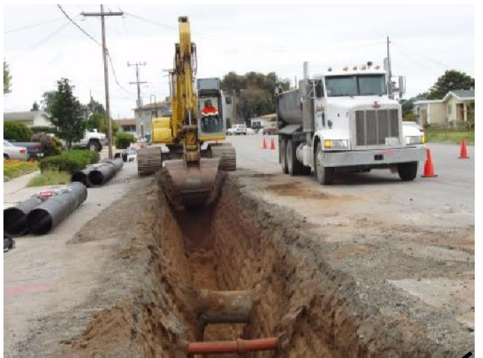
CRESCENT AVENUE CONSTRUCTION #4
