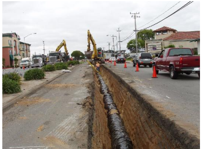
RESERVATION ROAD CONSTRUCTION #2
