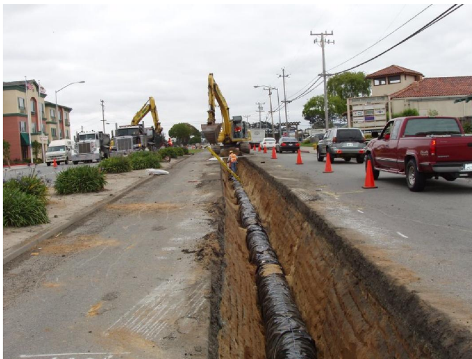
GENERAL JIM MOORE BOULEVARD CONSTRUCTION #3
